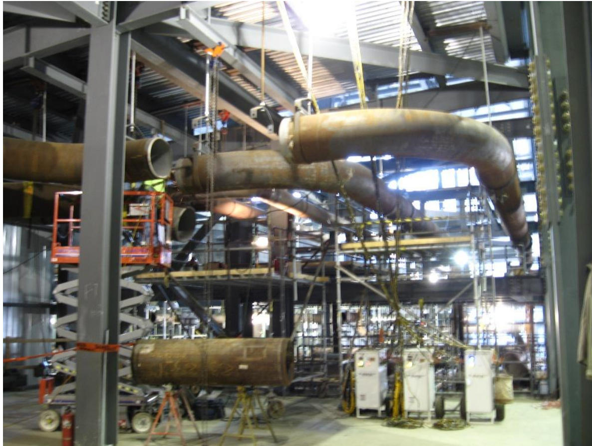
Steam Piping Construction
