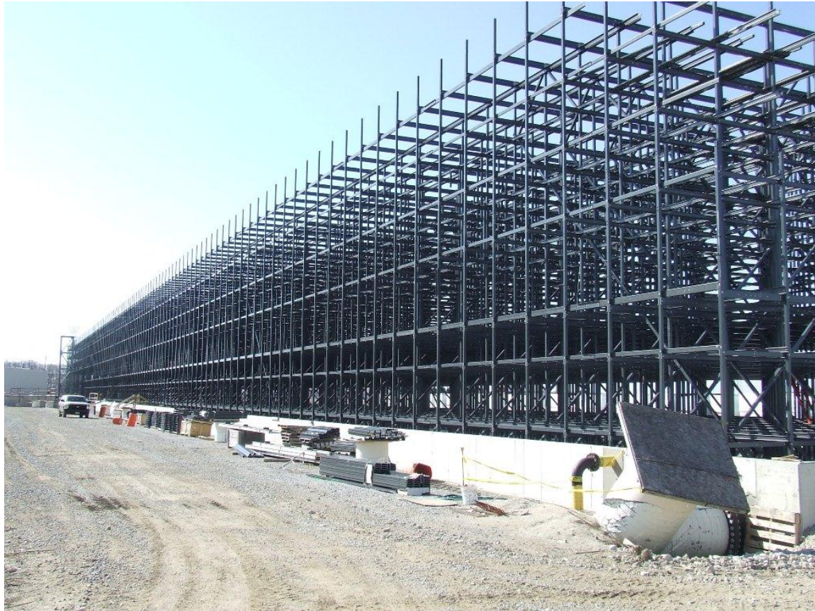
Cooling Tower Construction
