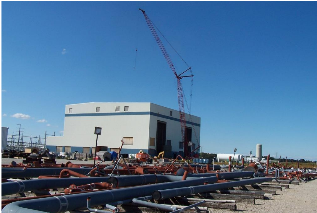
Laydown Area and Plant Building
