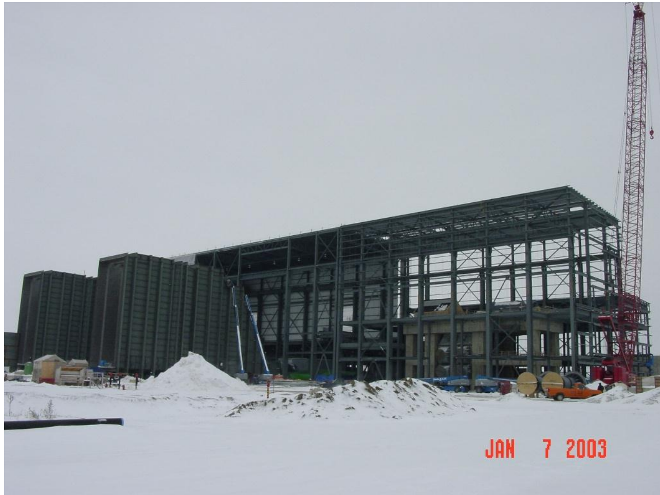
East Side of Plant in 2003
