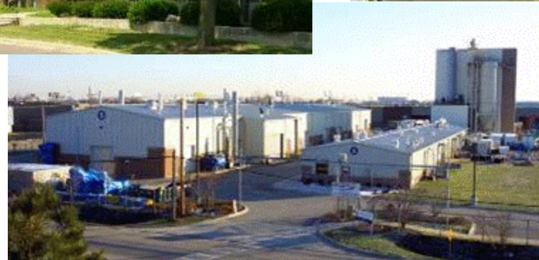
Energy & Environmental Technology Center
