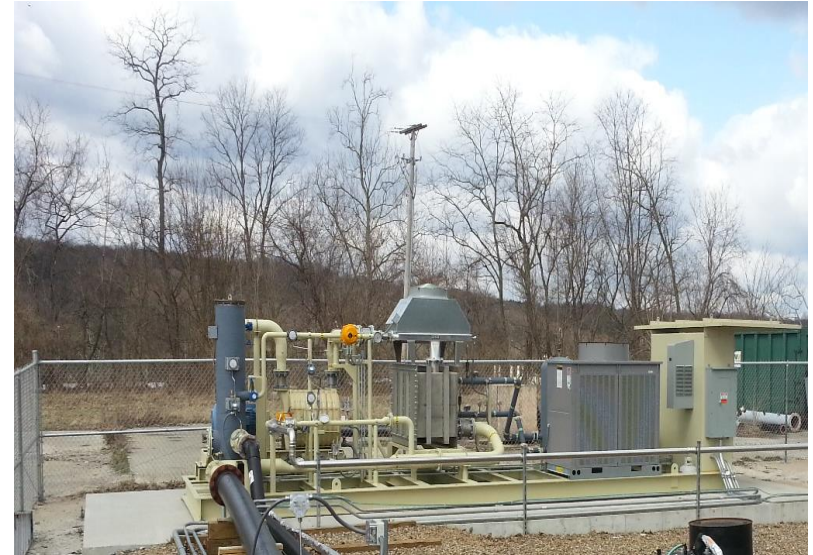
Hardy Road bio-gas conditioning and cleaning skid
