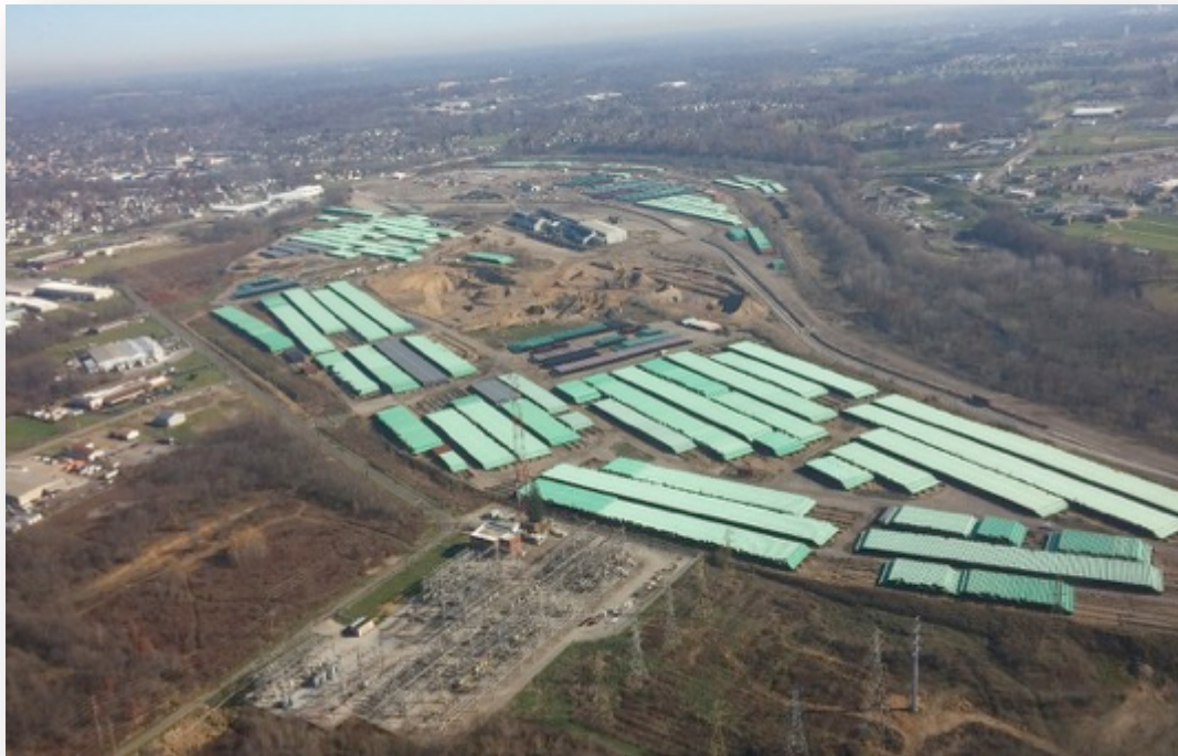
Photo: Over 700 miles (55,000+ pieces) of Rover pipeline located at Massillon, Ohio. The 500-acre site is the largest pipe laydown yard in North America.
